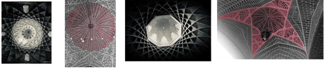
Figures 2-2” (a, b, c, d) Various ceiling decorations, including Karbandi, Rasmi Bandi, and Yazdi Bandi
