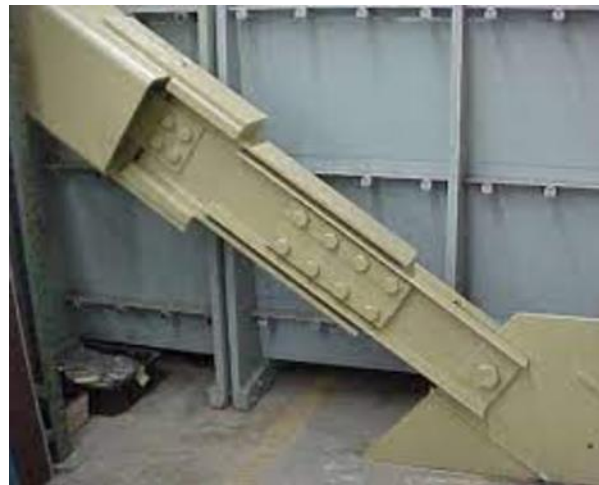
Figure 1. Pal Friction Damper Used in Diagonal Bracing
