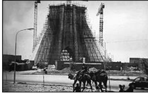
Figure 1. Azadi Tower during Construction (1970 / 1349 H.S.)
