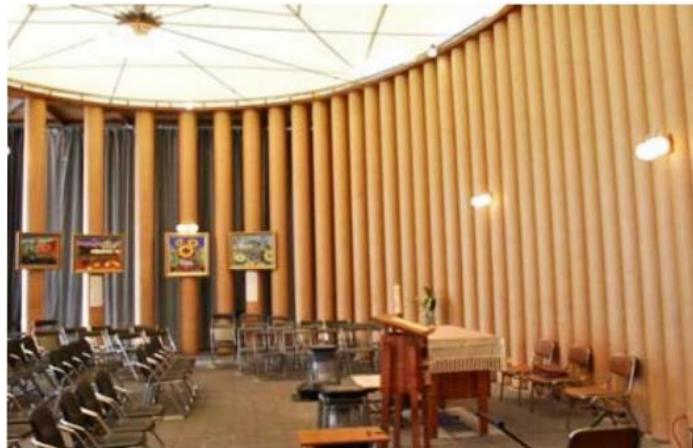
Figure 2. Installation of Paper Columns
