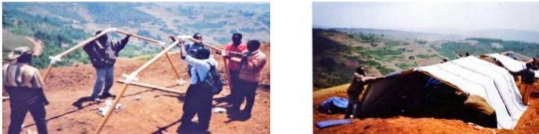
Figure 1. Emergency Shelter with Paper Structure (Shigeru Ban) for African Refugees and the Executive Details of the Paper Tube Frame in the Emergency Housing Phase.
