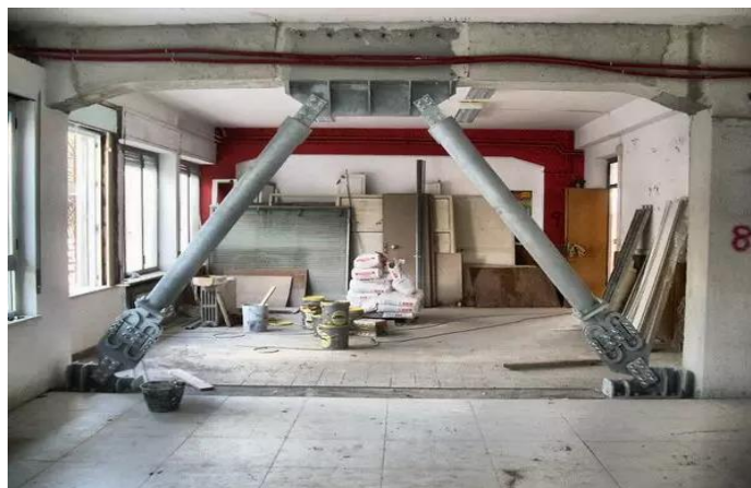
Figure 3: Strengthening with Steel Bracing (Source: Pourabdollah Ghadam, 2024)
