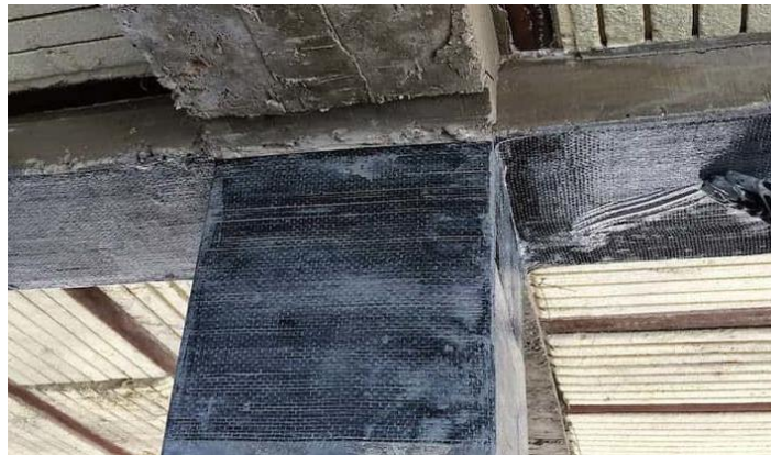
Figure 1. Strengthening of Columns and Beams with FRP
