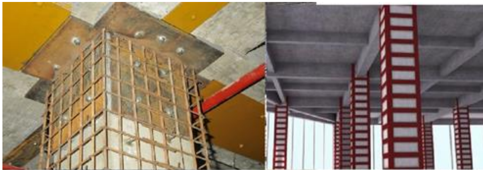
Figure 2. Strengthening with Concrete Jacketing (Source: Pourabdollah Ghadam, 2024)
